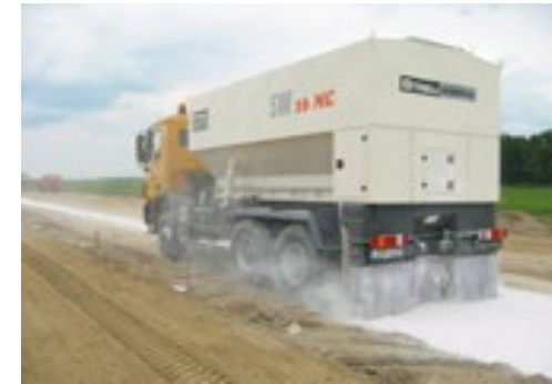
Cement spreader + our technology (mineral powder)
